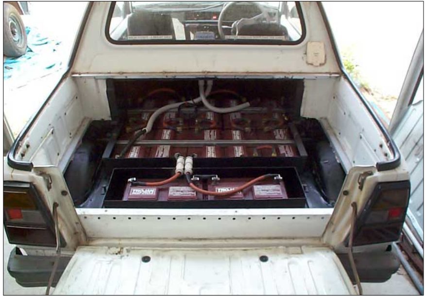
The batteries are mounted under the tray, so the cargo area is still fully useable.
